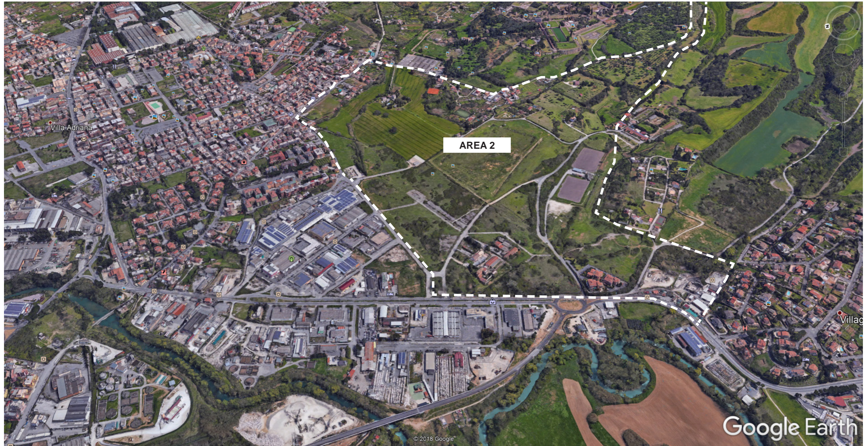
Bird's eye view with the perimeter of the area for landscaping (Area 2).
